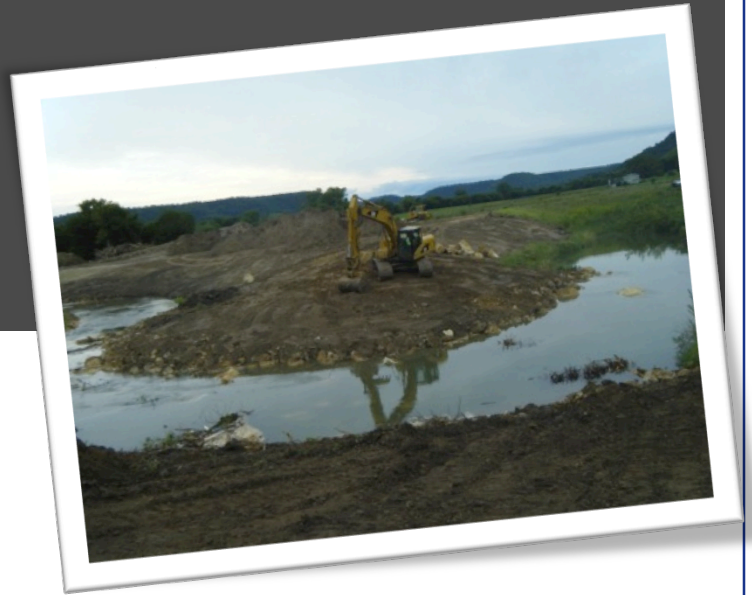
STREAM RESTORATION WORK CONTINUES ON COON CREEK NORTH OF COON VALLEY.
